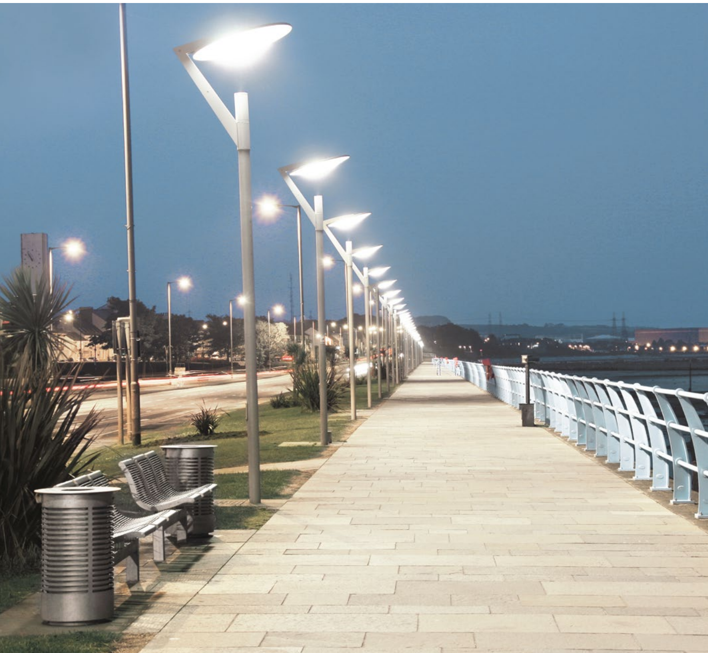
Modern street lighting with high reliability and long lifetime
