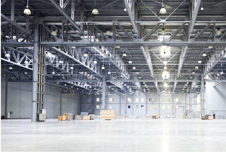
High bay application
